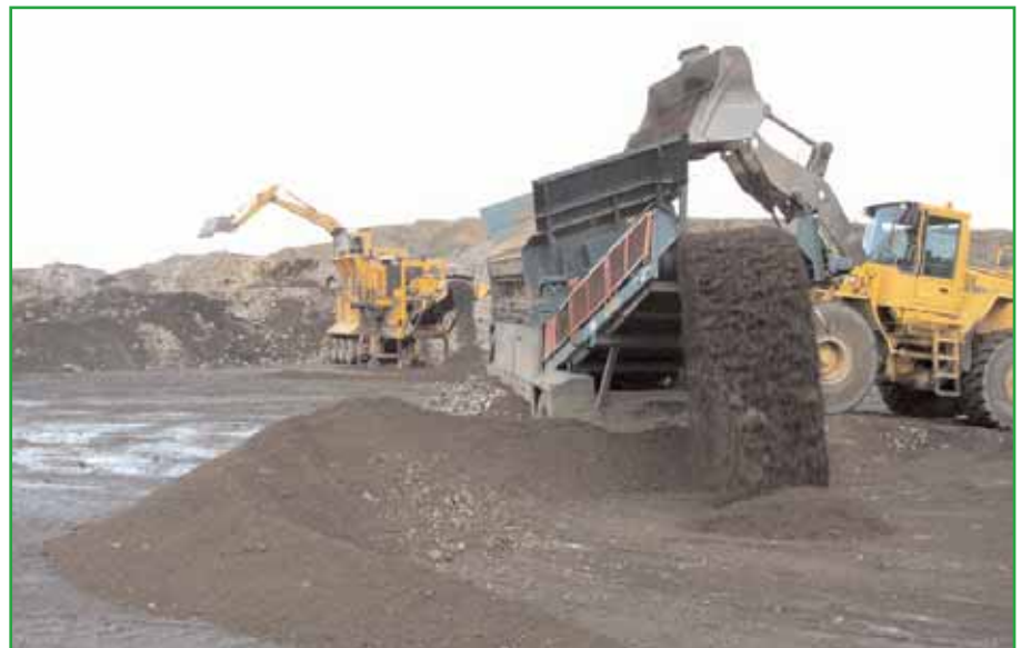
Recycled paving operation
